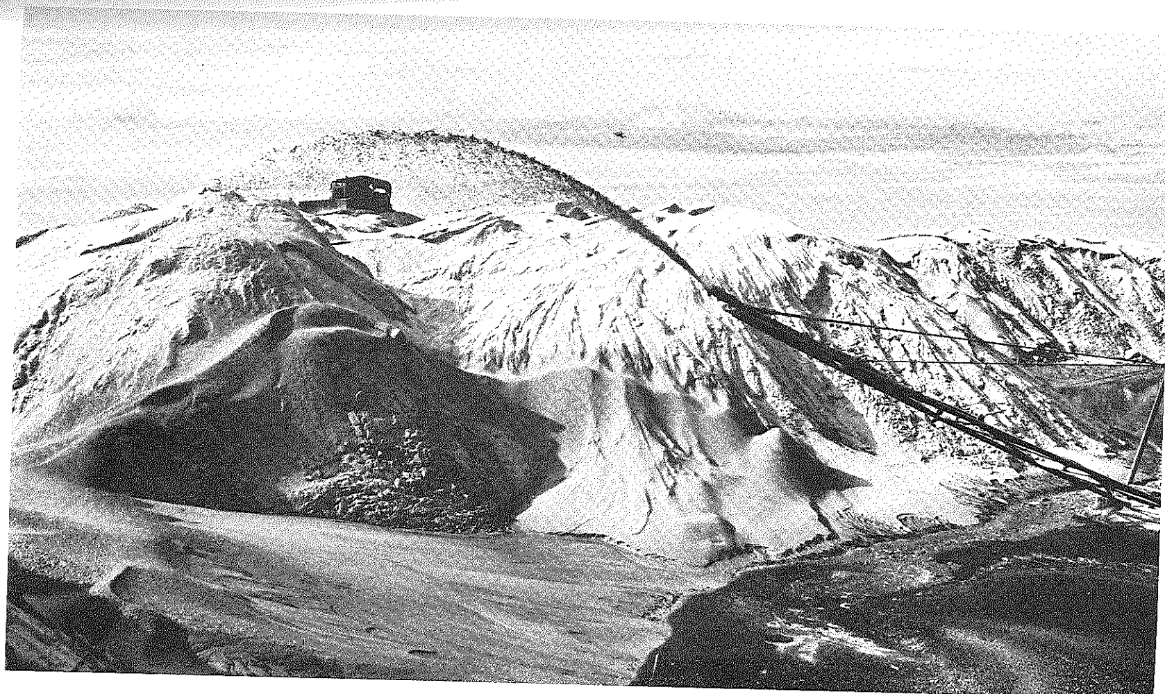
Tailings being placed behind the Queensland Titanium Mines Pty Ltd floating plant
